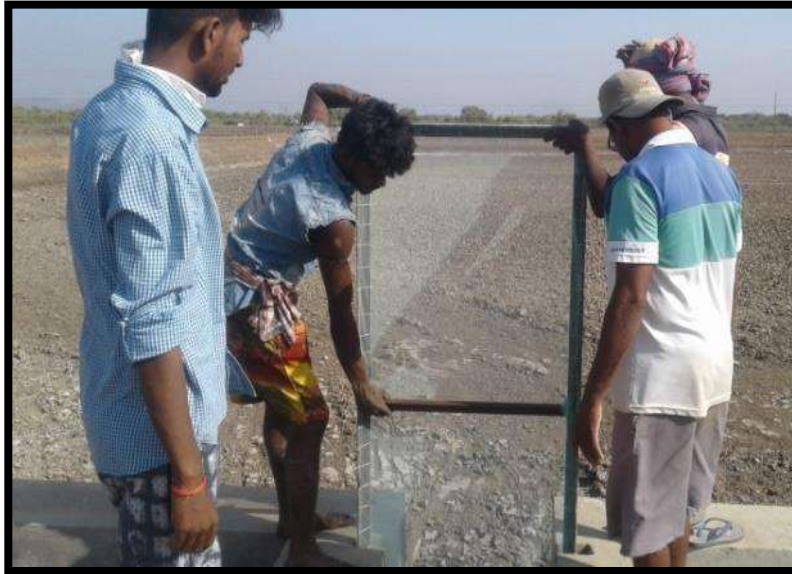
PACKING OF THE SLUICE GATES ON DATED 22 FEBRURY 2019
